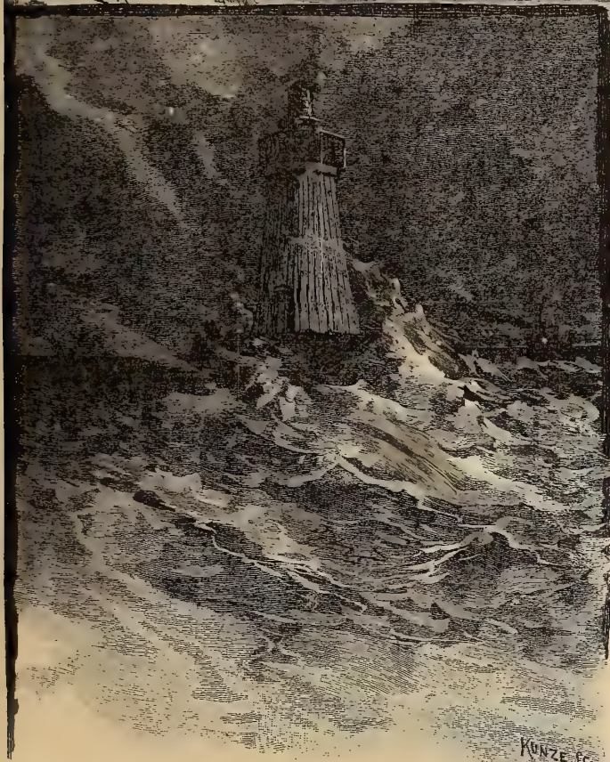
PIER END LIGHT.
